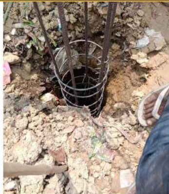
REINFORCEMENT CAGE
